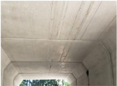
Photo 3: Culvert barrel soffit
