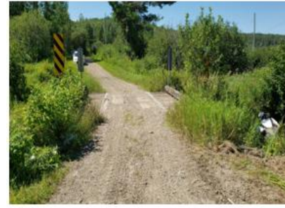
Photo 1: Structure from south approach
