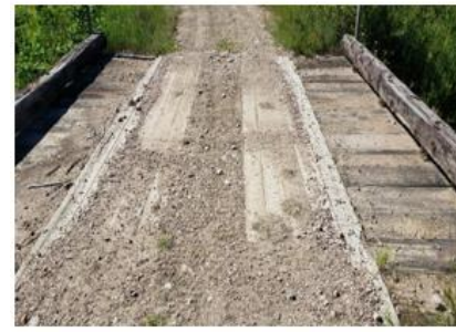
Photo 3: Deck wearing surface
