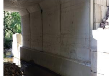
Photo 6: West abutment wall
