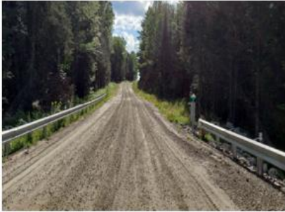
Photo 1: West approach from centre of structure
